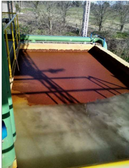
Ferric Chloride Floc with Arsenic Retention
